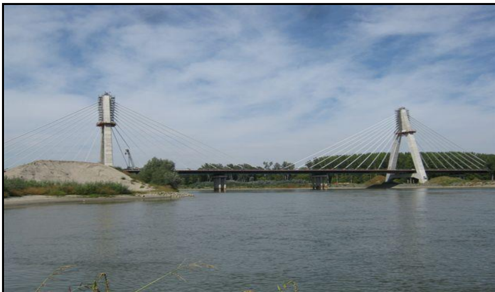
Figure 5: View of the Drava Bridge in the construction phase
